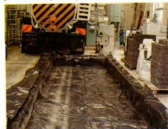
Fig 1. NUROLF test site showing waterproof material prior to installation of crushed rock open graded roadbase.
