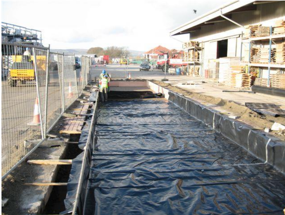
Figure 9. 2000 gauge polythene was installed to achieve tanked conditions for each Test Item.
