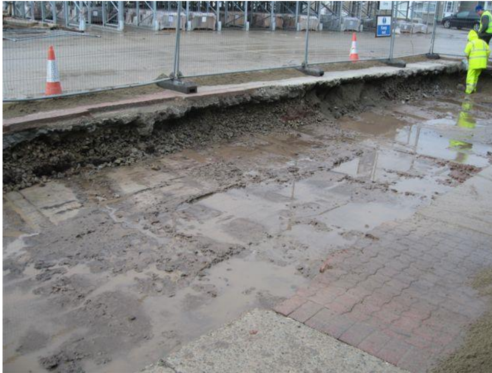
Figure 7. The test area has been excavated to reveal alluvium clay with a California Bearing Ratio of 5%.
