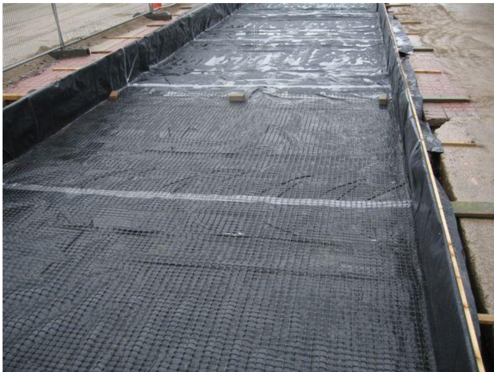
Figure 10. Test Item 4 required the installation of two layers of a geogrid material known as Tensar SS40. The lower layer is shown here directly over the polythene membrane.
