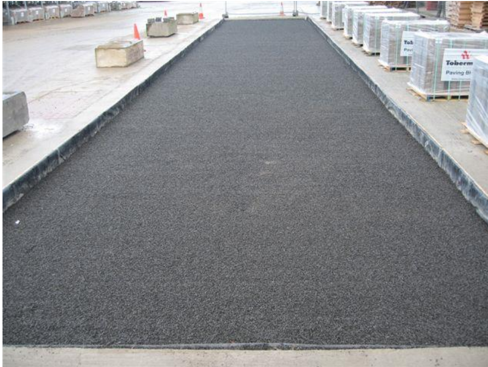
Figure 11. Prior to the laying of pavers, a 50mm thick course of 6mm single sized grit was installed in each Test Item.
